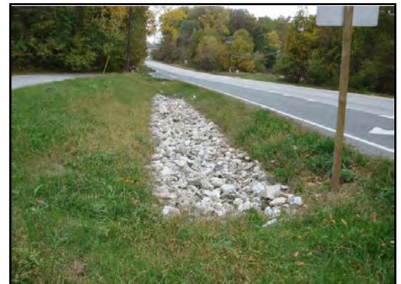
**Infiltration trench with exposed stone; must drain in 48 hrs**
