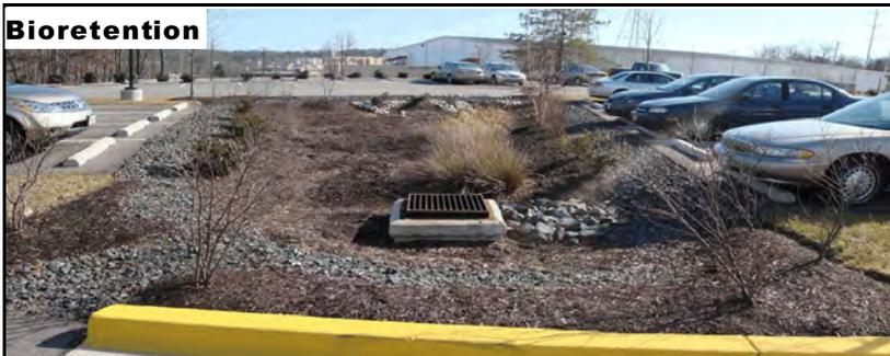
**Minimum 6 inches storage, 2-3 inches mulch; must drain in 48 hrs; wetland plants indicate poor drainage, failure**
