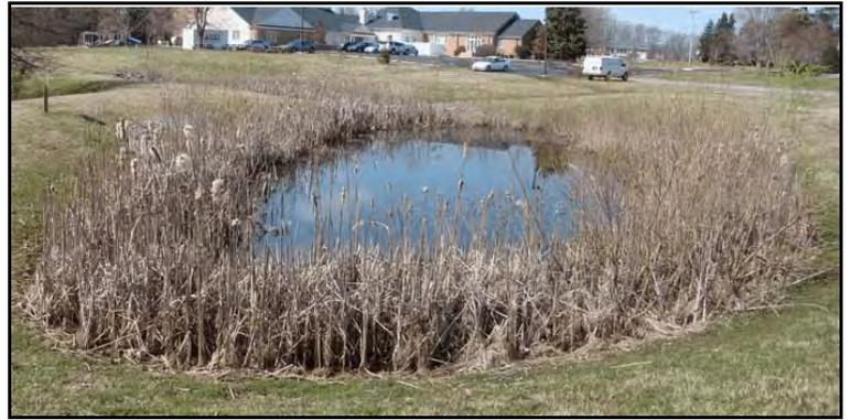
**Pond must be cleaned to original capacity when half- full of sediment, cattails or other plants**
