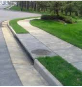
Storm Drain Inlet
