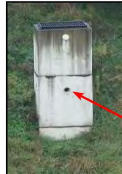
**Infiltration basins** must hold runoff until it can soak into the sandy soils of the basin floor so the spillway usually lacks an opening until a foot or two above the floor.
