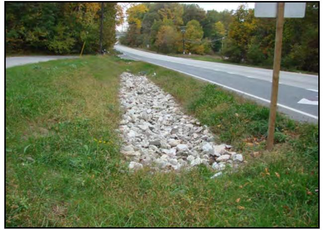
**Infiltration Trench (IT)** Stone or gravel usually exposed at surface often with observation well
