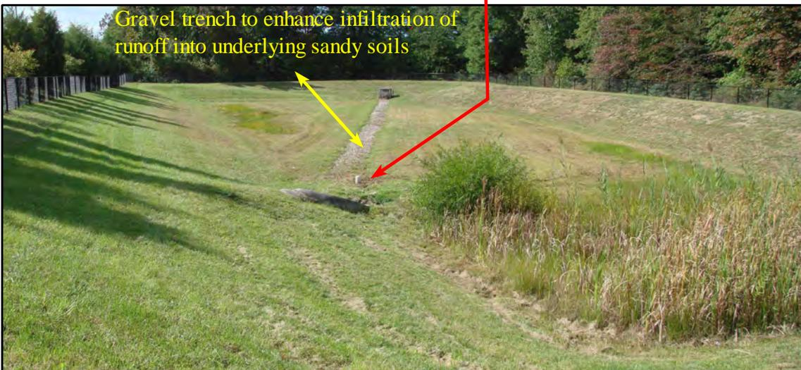
Gravel trench to enhance infiltration of runoff into underlying sandy soils
