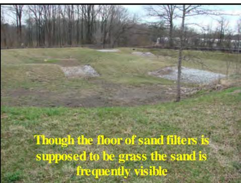
Though the floor of sand filters is supposed to be grass the sand is frequently visible
