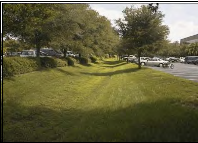
Dry (Bio) Swale
