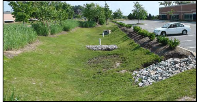
Bioretention with Grass
