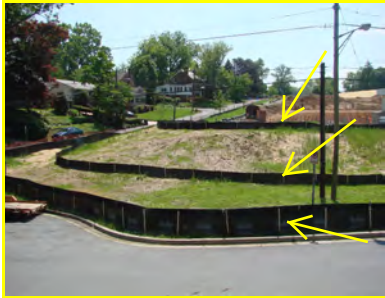
Perimeter Silt Fence Rows
