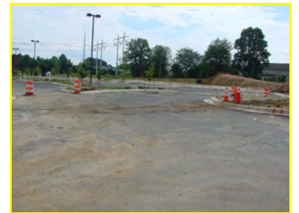
Paved parking lot
