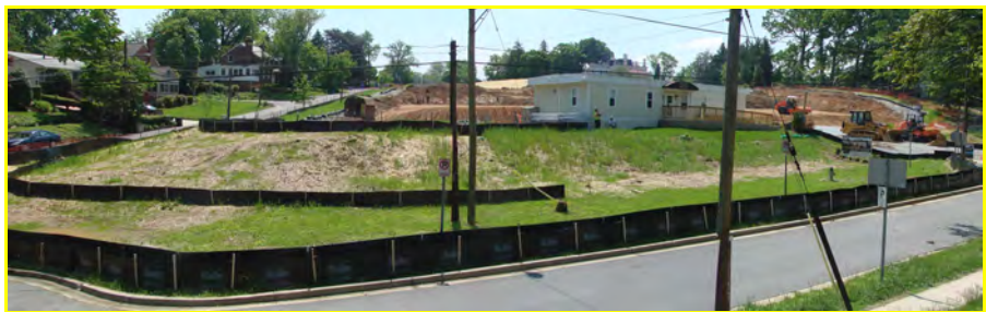
Silt Fence & Earth Berm
