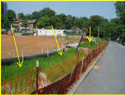
Perimeter Earth Berm With 95% Grass Cover
