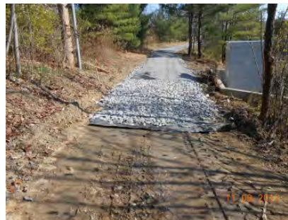
Road bed stabilized with stone
