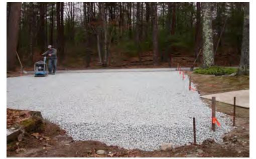
Parking lot stabilized with stone
