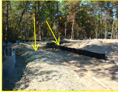
Silt Fence & Earth Berm
