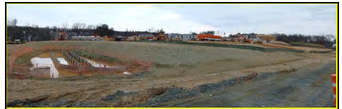
Full Stabilization Required At Rough Grade
