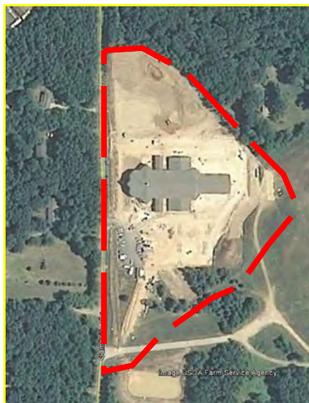
Interior Has Been Cleared: Nonerodible Areas (Building + Lower-Left Parking) = 30% of site; Of The Pervious Areas 90% is Exposed Soil
