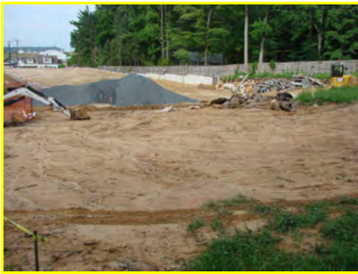
Fully exposed soil between stone pile and grass
