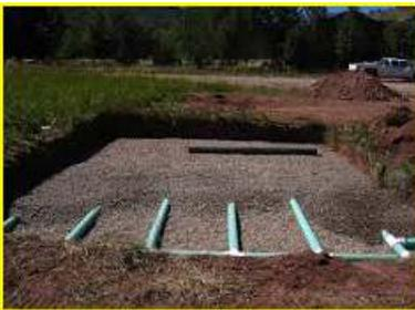
On the other side of this factsheet you'll find a typical sand filter design from the [Maryland Stormwater Design Manual](#). As shown to the left, a pit is excavated. A gravel drainage layer is placed on the bottom. Perforated plastic pipes are then placed on the gravel. More gravel is added to cover the pipes. This is then covered with two- or three-feet of sand. The filter should hold water no more than a day or two after each storm, thus negating mosquito problems.
