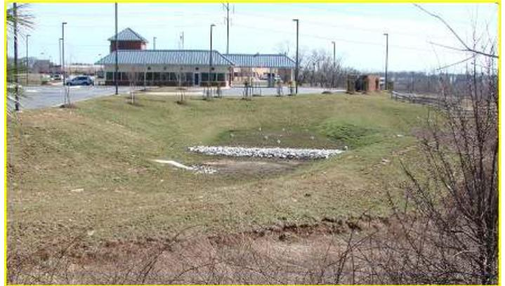
As the name implies, this BMP filters pollutants as stormwater runoff infiltrates through a two- or three-foot layer of sand. Sand filters are moderately effective measures for keeping stormwater pollution out of nearby waterways. The filters are usually constructed on sandy or other permeable soils. But with an underdrain a sand filter can be installed on any soil.
