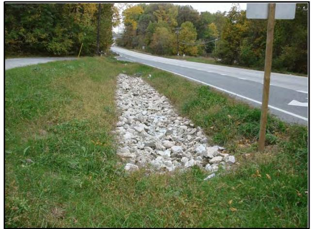
**Infiltration Trench With Exposed Stone**
