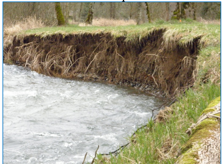
Severely eroded banks make walking dangerous
