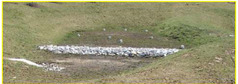
Numerous white PVC caps are frequently present in a sand filter
