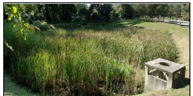
Wet Pond: Full of Cattails; No Storage Remaining
