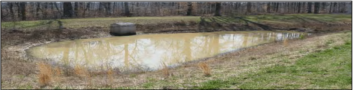
Wet Pond: Full Capacity; Little Sedimentation
