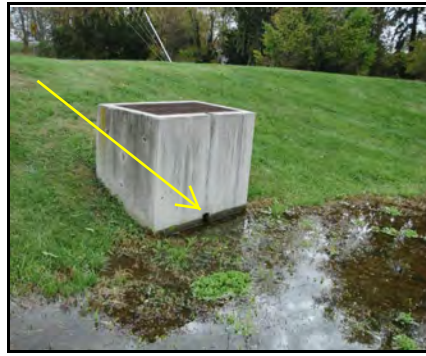
Dry Pond: Opening At Riser Bottom
