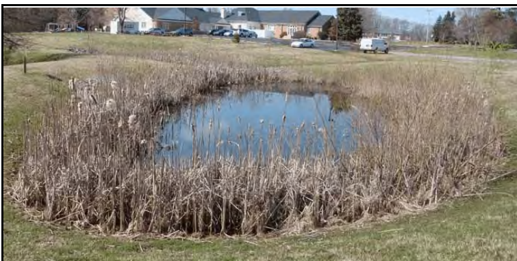
Wet Pond Partially Full With Sediment-Cattails
