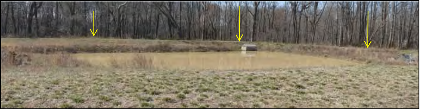
Straight, Level Earth Embankment; No Low Spots; No Trees or Burrows on Embankment
