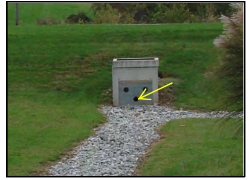
Infiltration Basin: Opening Above Riser Bottom
